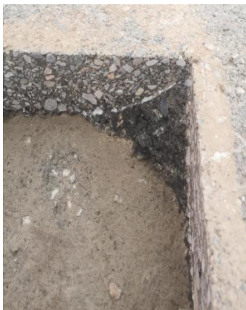
①坑槽开挖
